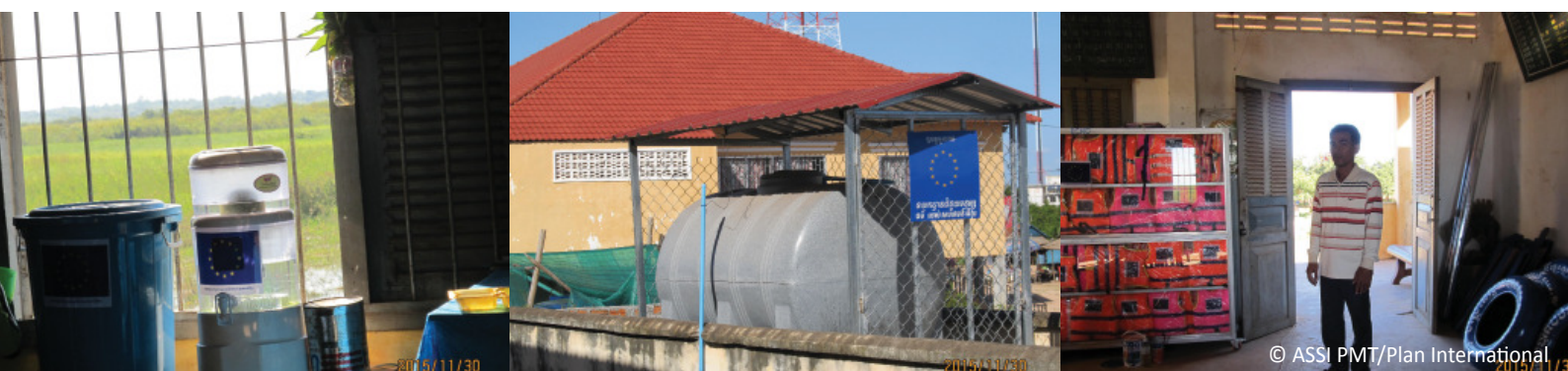
Water filter and water reservoir identified to minimize the hazards
