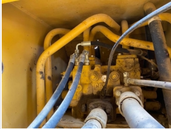
Appearance of Hydraulic Lines / Fittings Photos
