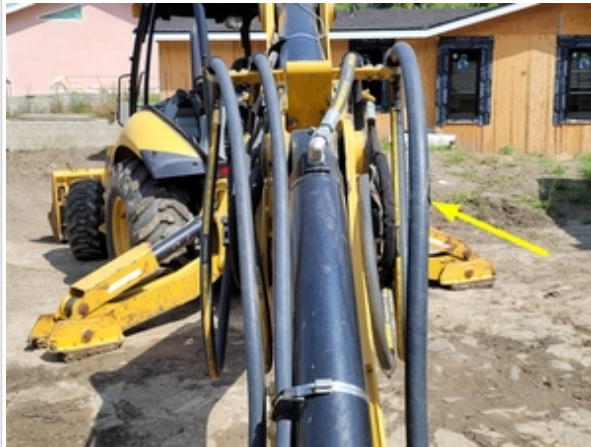
Minor hose damage to auxiliary hose
