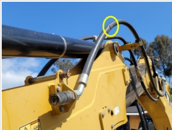
Minor hose damage
