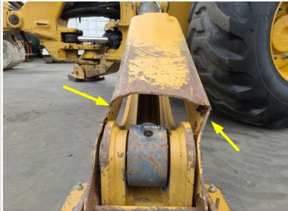
R/S Stabilizer Cylinder Guard Bent
