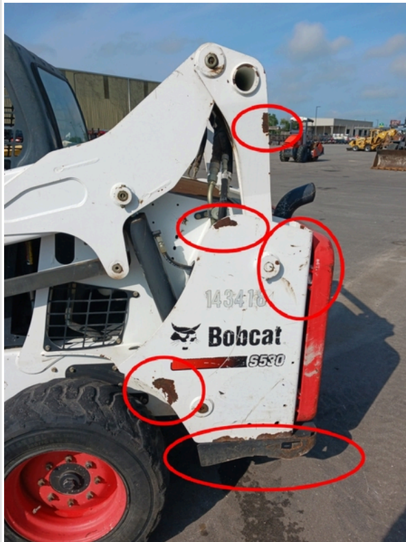
areas of rust and missing paint and there is a dent on the left hand side behind the left rear tire
