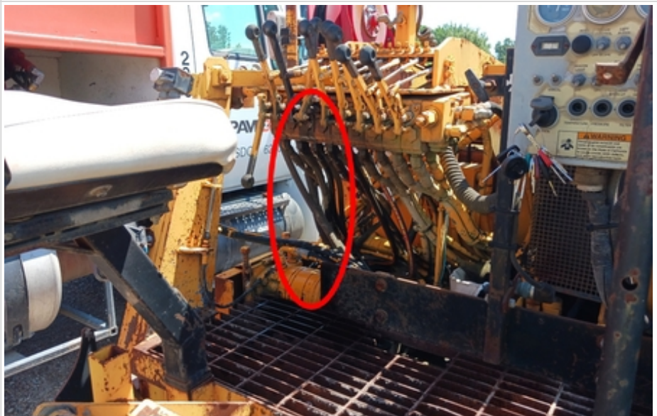
left side lever control panel is leaking hydraulic fluid
