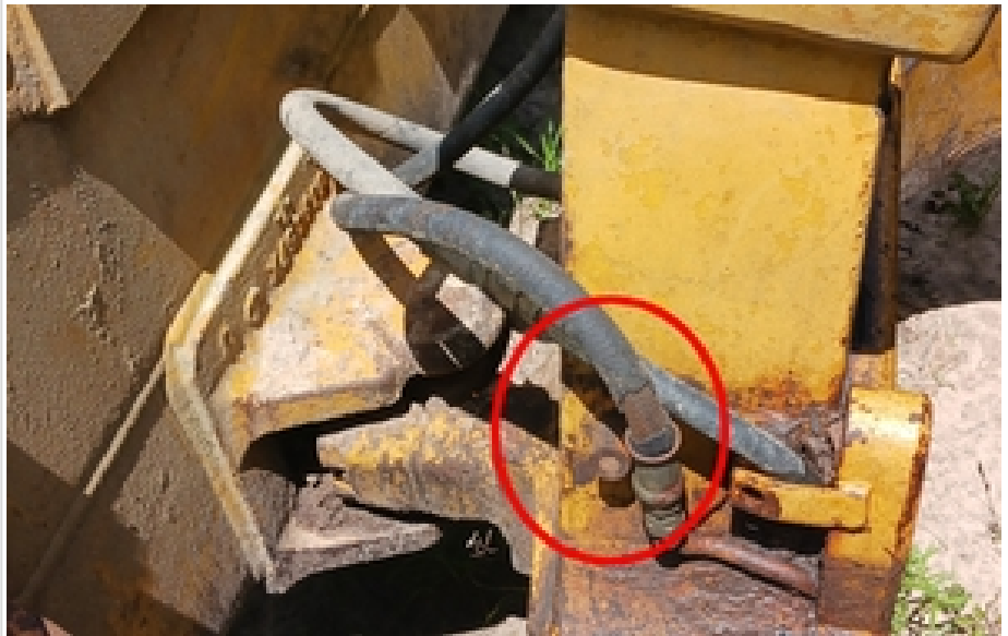
old cracked hoses
