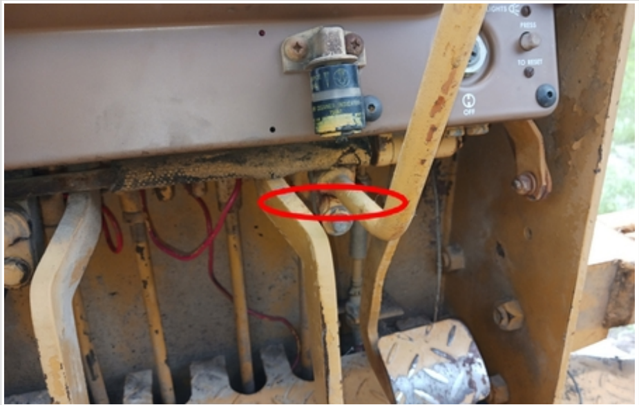
area is cracked down the middle, causing control levers to move side to side
