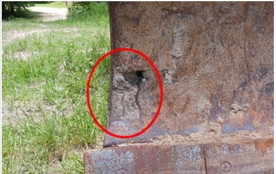
damaged area on blade
