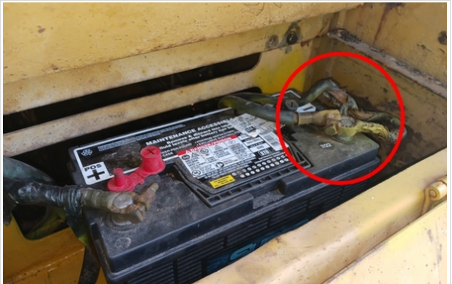
exposed wires on negative battery cable
