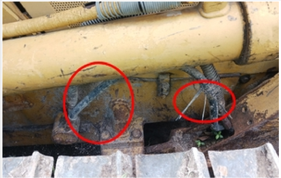
dry/cracked hose and zip tied hoses
