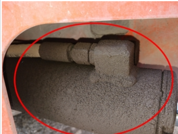
damp dirty area
