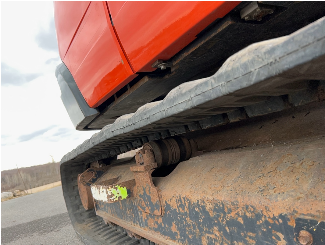
Right Track Condition / 03-27-2024
