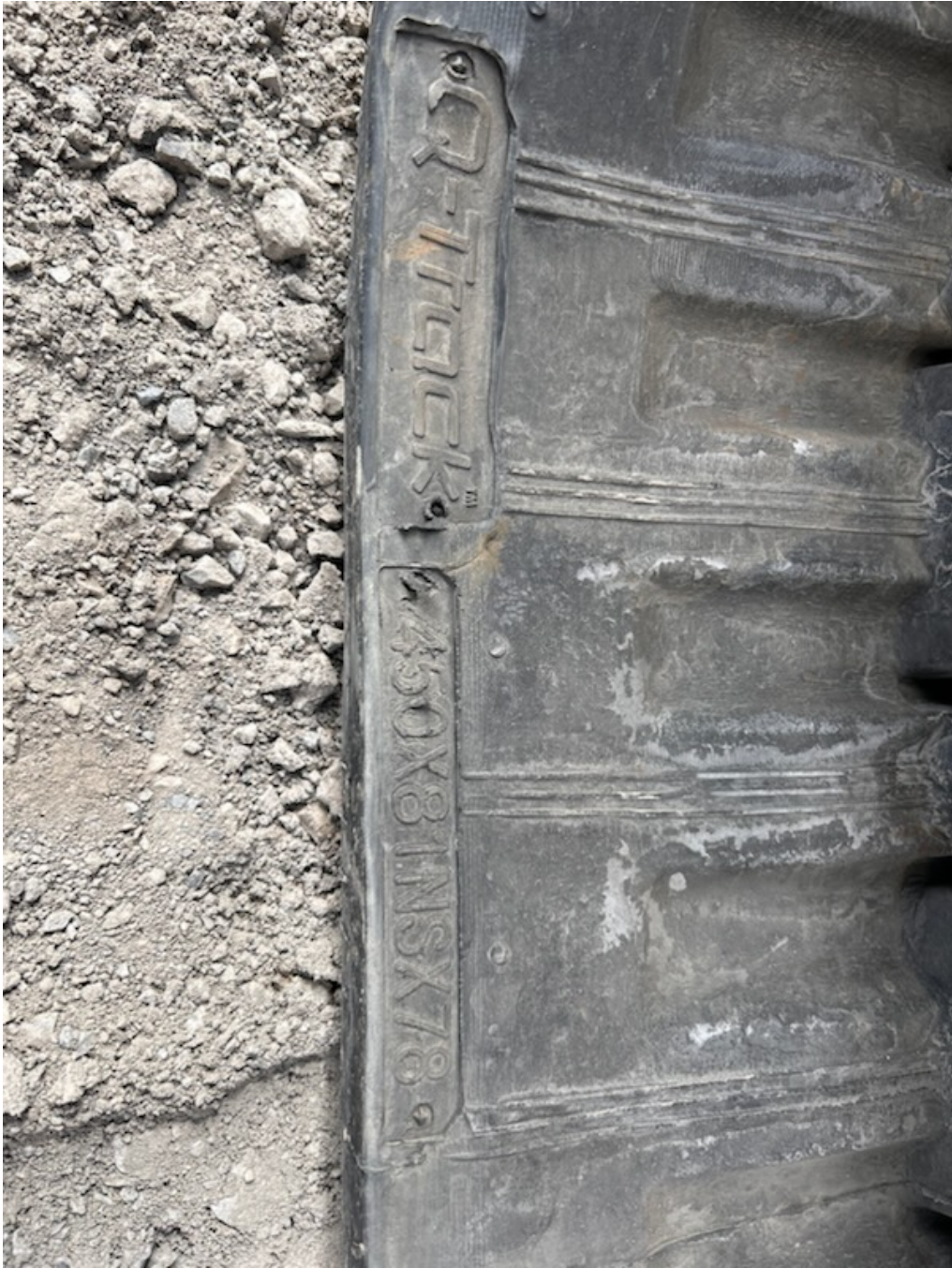
Left Track Brand / Left Track Size / 03-28-2024
