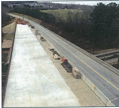
The Bill Carruth Parkway Bridge widening finishes next summer.
