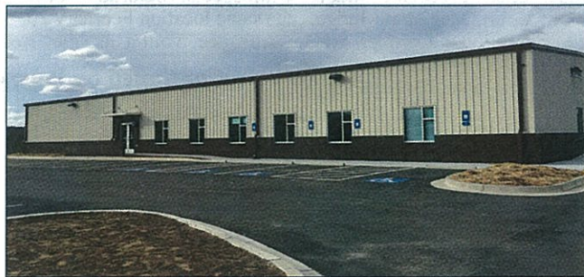
The new Paulding Sheriff's Officer Training Center accommodates various sizes and types of classes.
