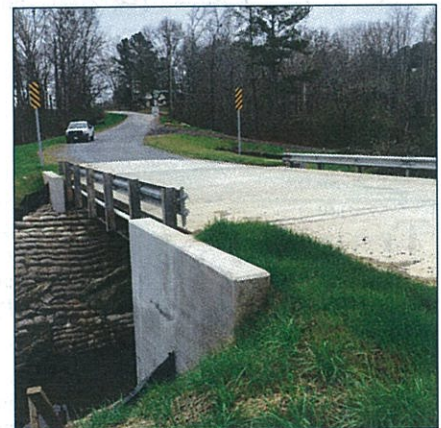
2015 bridge work included this one on Lee Road, completed in October.
