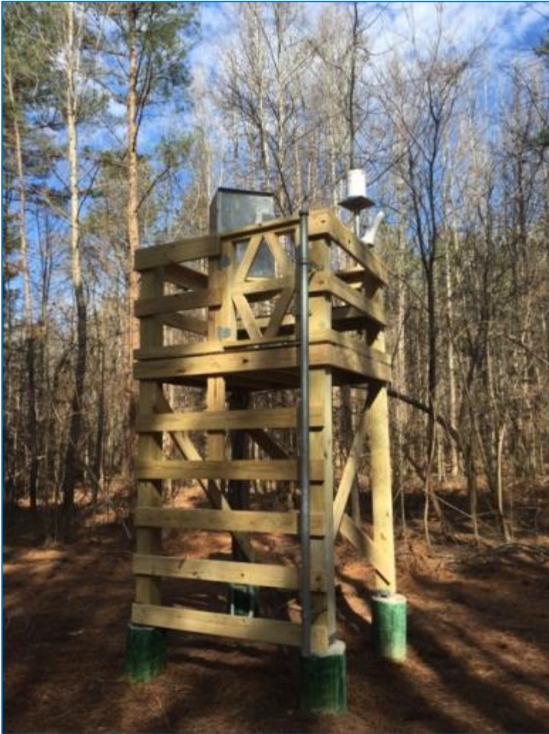
Elevated Monitoring Station Tower
