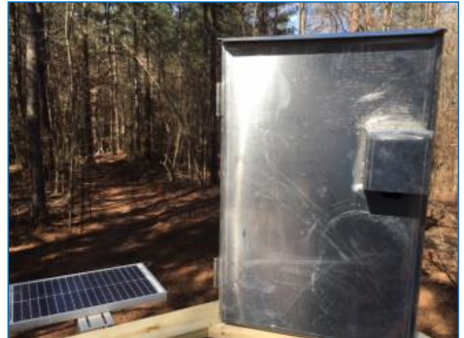
Instrumentation Enclosure and Solar Array
