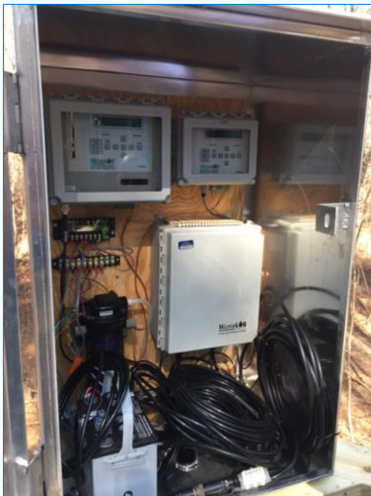
Instrumentation Within Secure Enclosure
