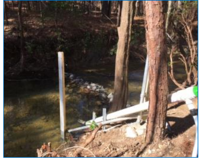
Gage and Probe Installation in Richland Creek
