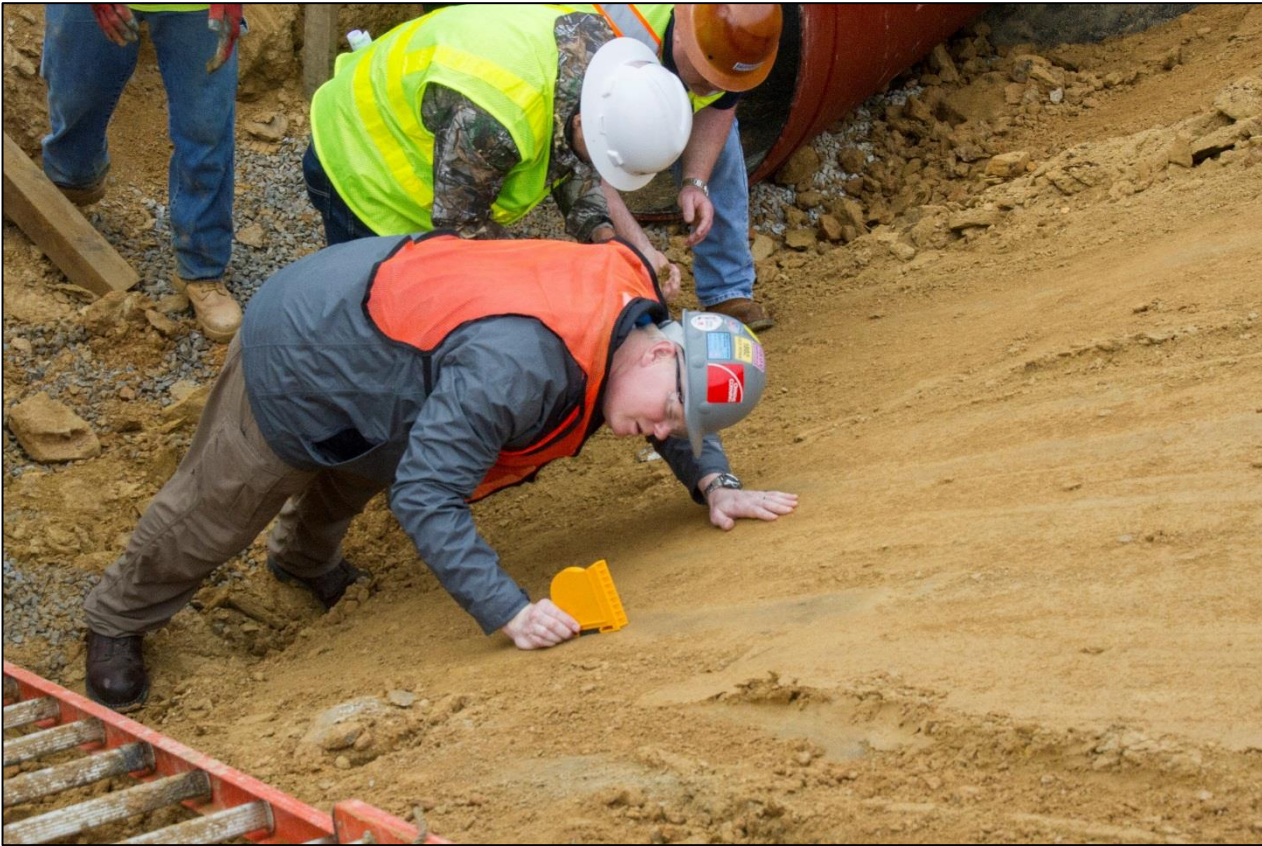
Measuring the slope of a trench
