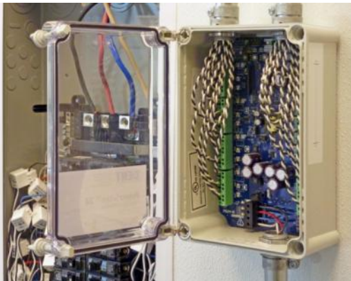
PowerScout 24 mounted in a NEMA-rated box near electrical panel
