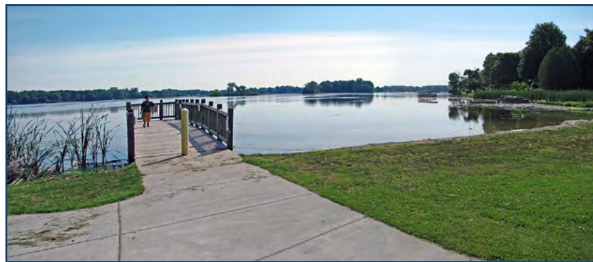
Existing dock/pier, Lakeside Park
