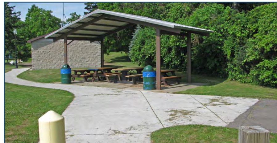
Picnic Shelter, Lakeside Park
