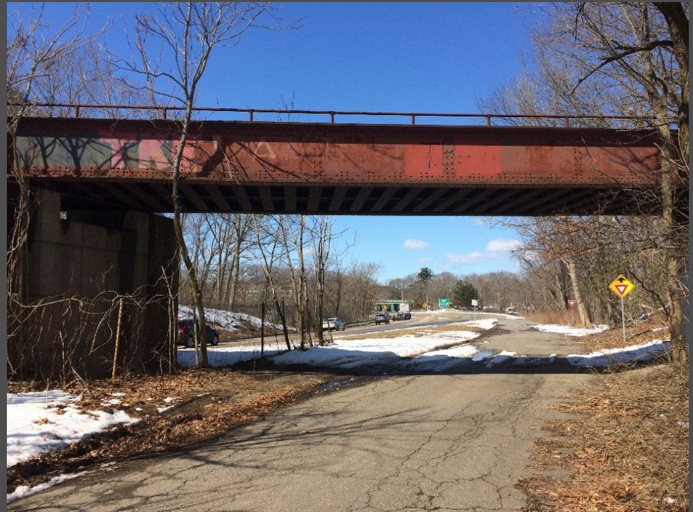
One of two former rail bridges over I-95
