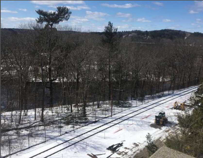
The Rail Spur in March 2019
