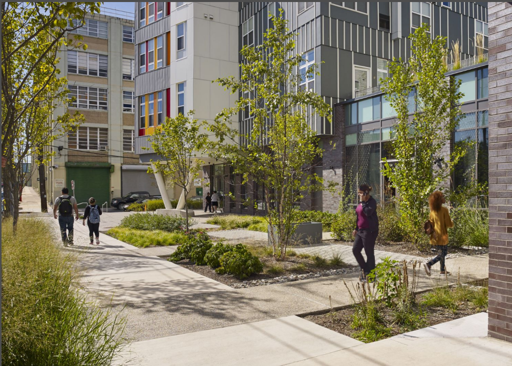
Paseo Verde in Philadelphia, PA is a LEED Platinum mixed-use transit oriented development with 120 units of mixed-income housing (1-3 bedroom units; 53 units or 44% are subsidized).
