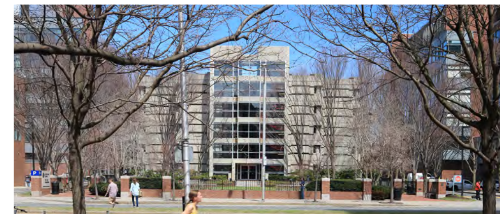
Existing Site Photo
