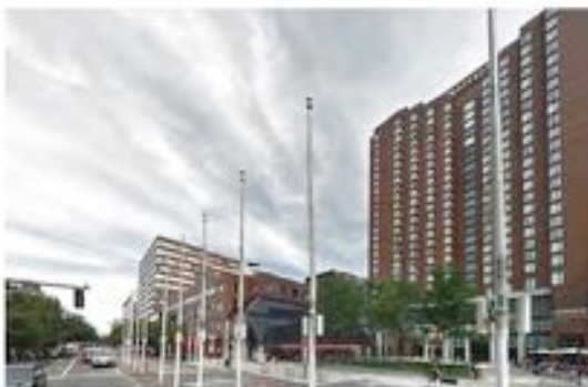
Existing Site Photo
