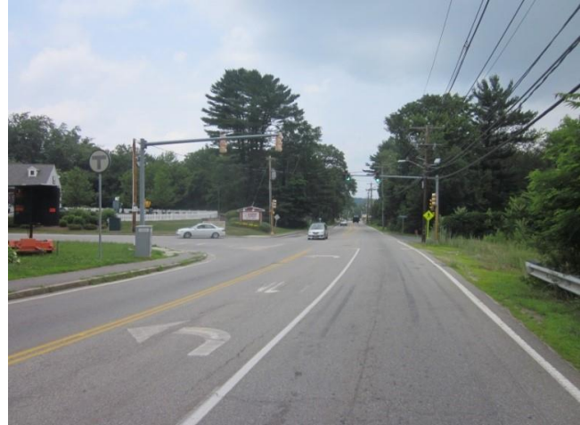
Looking northeast toward MBTA Access Road/Voyagers Lane
