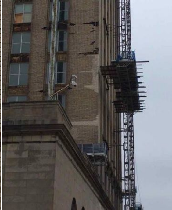
Tower brick replacement, northwest corner.
