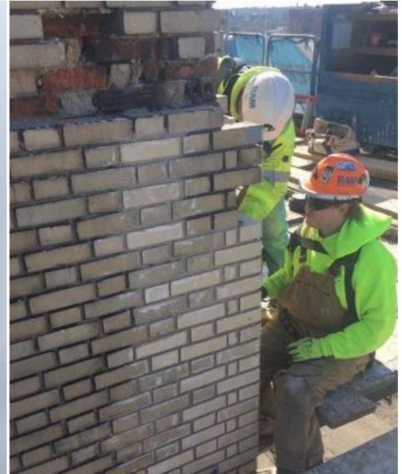
Tower brick replacement, southwest corner.
