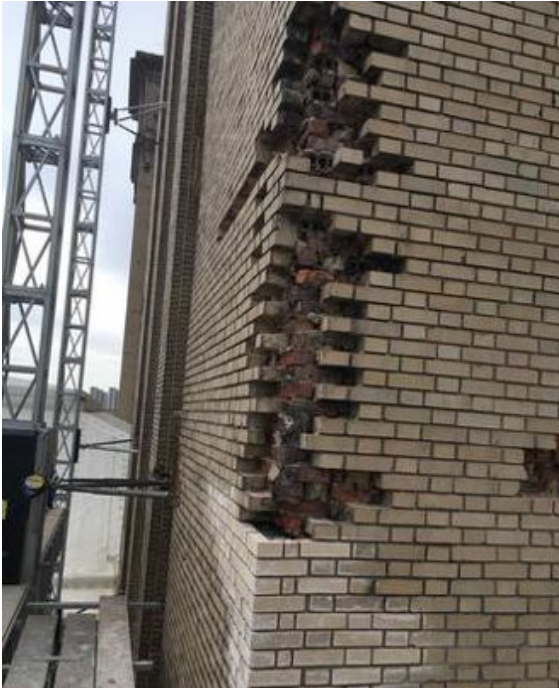
Tower brick replacement, north elevation west corner.
