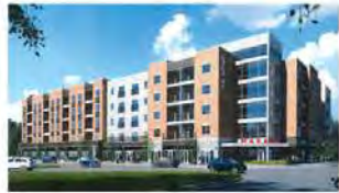
1 HI Vine: 5 story, under construction, 12,580 SF Retail, 73 Apts, 117 Beds.
