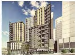
3 HUB Plus: 11 Story, under construction, 12200 SF Retail, 340 DU, 608 beds.
