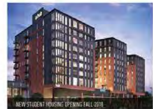
5 HUB on Campus: 11-stories, under construction, 1800 SF Retail 289 DU, 599 beds.
