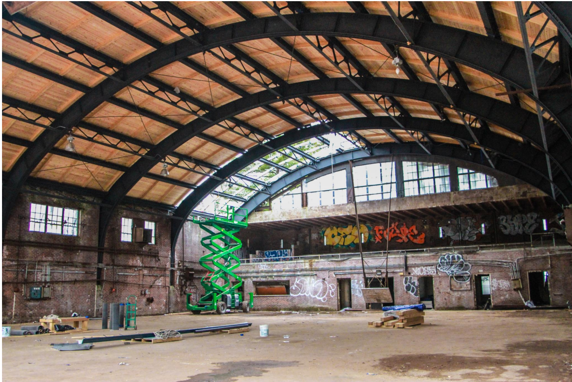
Restoration in Progress - Drill Hall, view West
