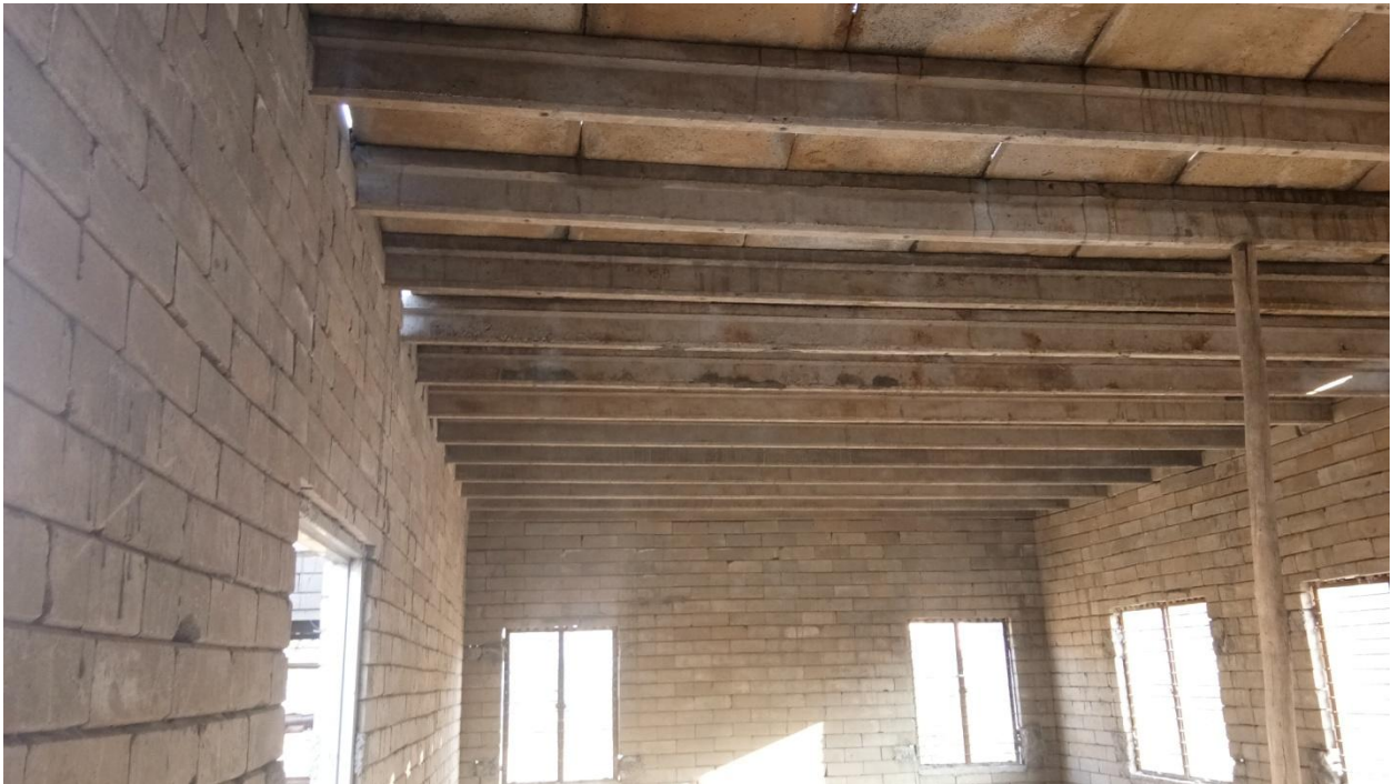
JOIST AND PAN PLACMENT FOR ROOFING
