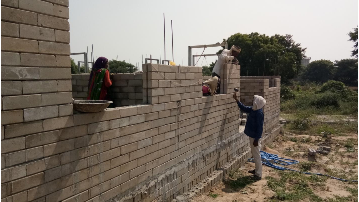
WALL CONSTRUCTION ACTIVITY
