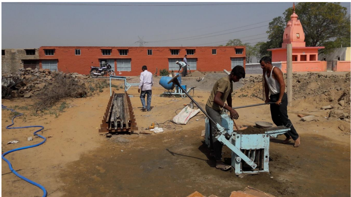
CIB & JOIST MANUFACTURING ACTIVITY AT GRAMALAYA
