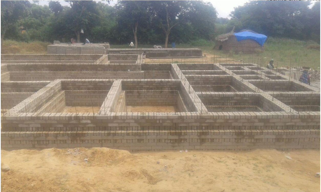
FOUNDATION OF THE GRAMALAYA
