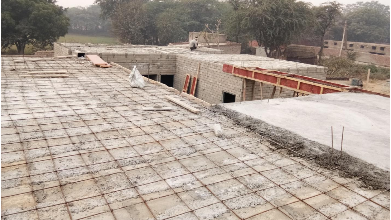
ROOF CASTING
