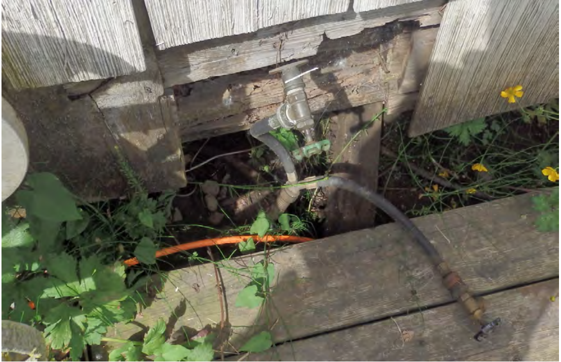
Photo 1.10: Unsafe condition - plumbing
