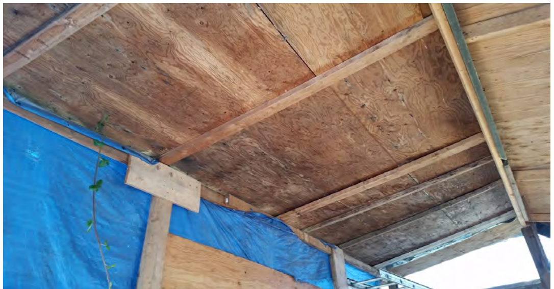
Photo 1.2 Addition without a permit – Structurally unsafe
