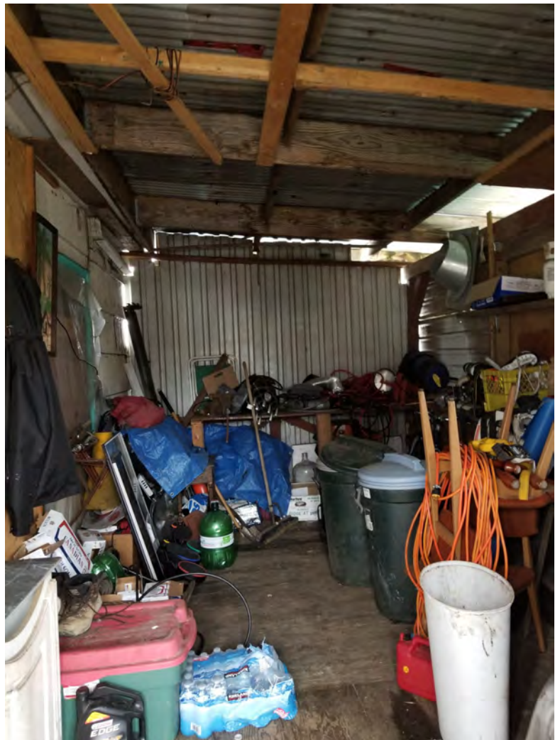
Photo 1.6 Addition without a permit – Structurally unsafe (interior)
