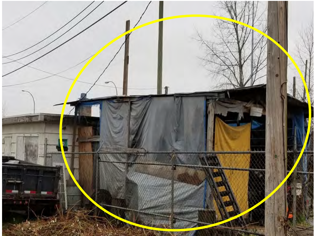
Photo 1.1 Addition without a permit – Structurally unsafe
