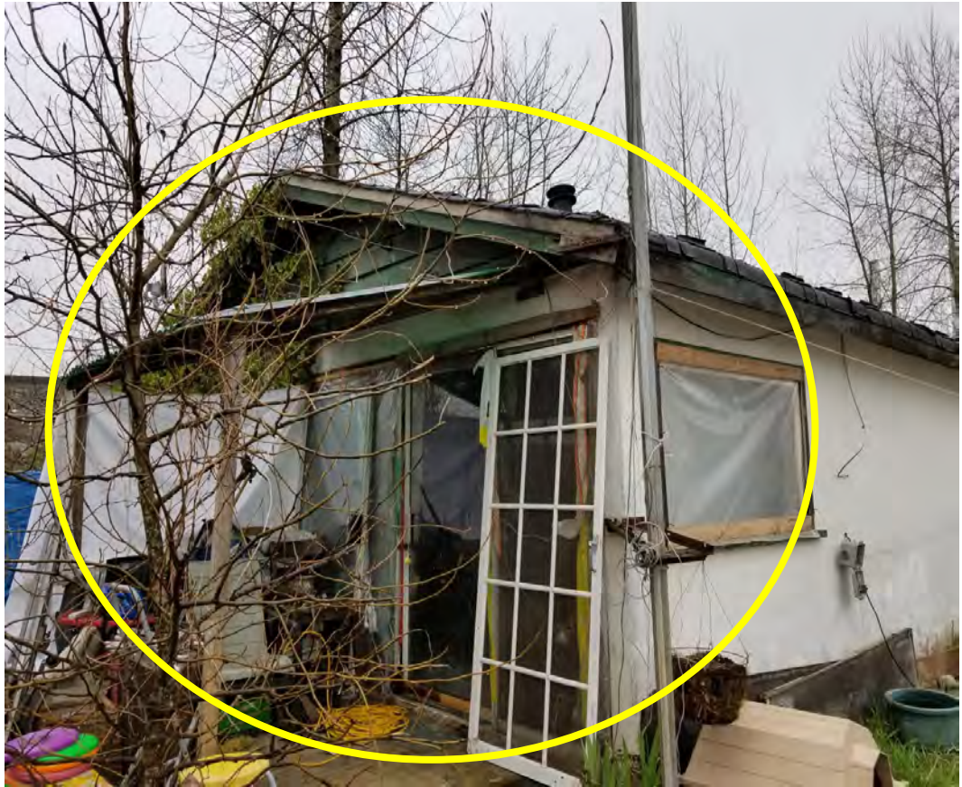
Photo 3.2: Addition without a permit – Structurally unsafe
