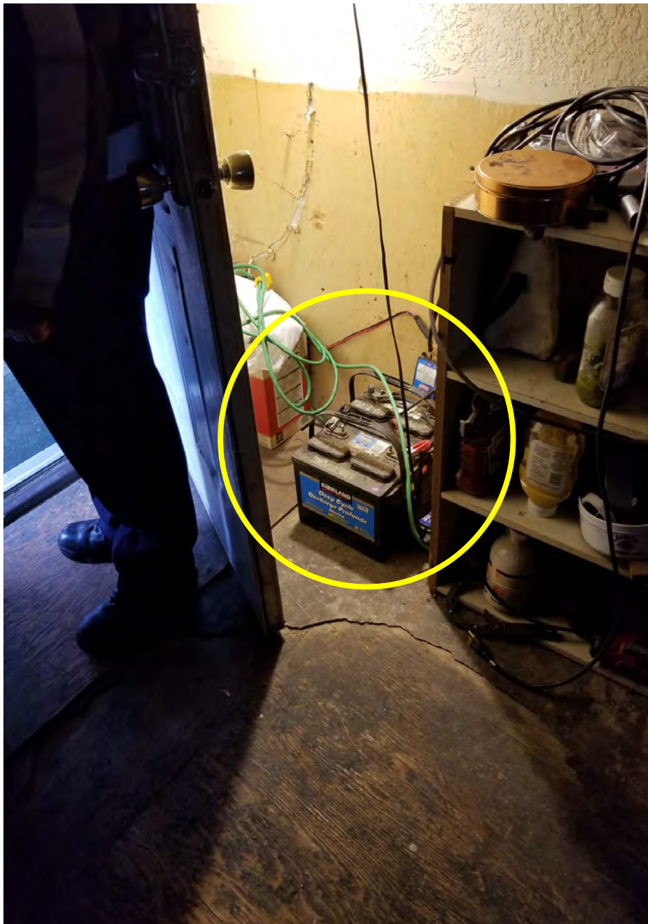
Unsafe condition – electrical
