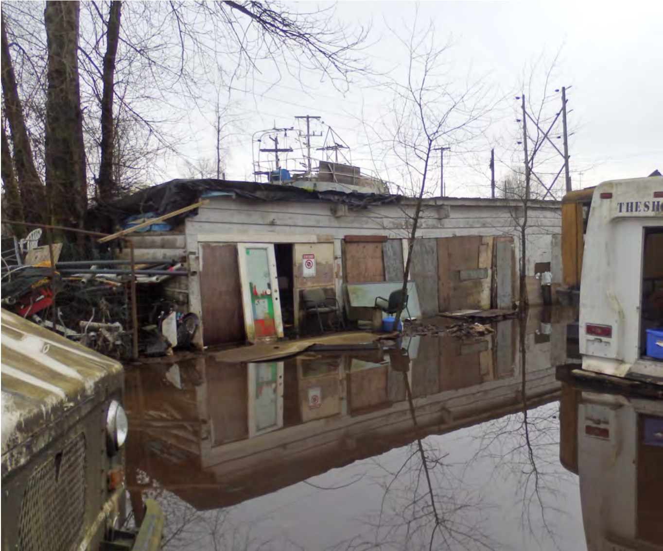
Photo 2.1: Unsafe building condition
