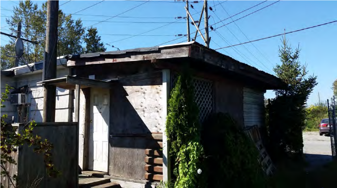
Photo 1.4 Addition without a permit – Structurally unsafe
