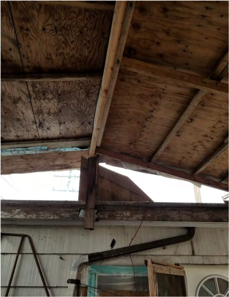
Photo 1.3 Addition without a permit – Structurally unsafe
