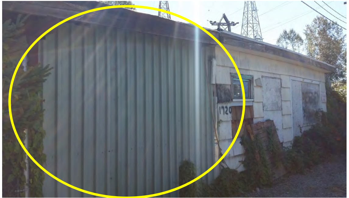
Photo 1.5 Addition without a permit – Structurally unsafe (exterior)
