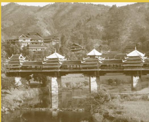
Dong "wind and rain bridge." PHOTO BY ARIAL STEINER.
