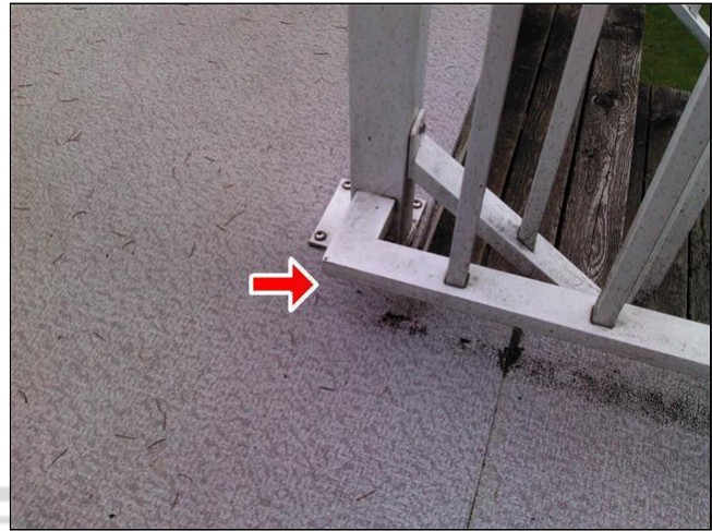
Handrails loose
