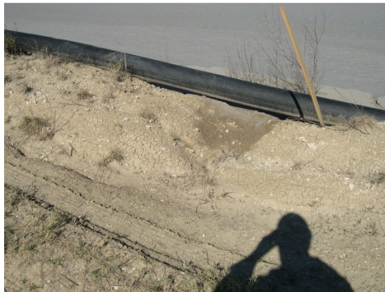
Figure 15: Erosion Gully
