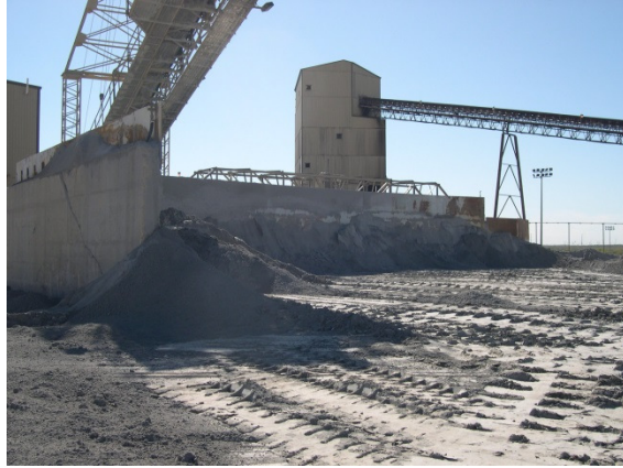
Figure 21: FGD Sludge Pile
