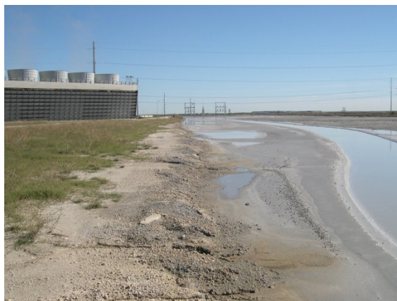
Figure 12: Wind/Wave Erosion Gullies
