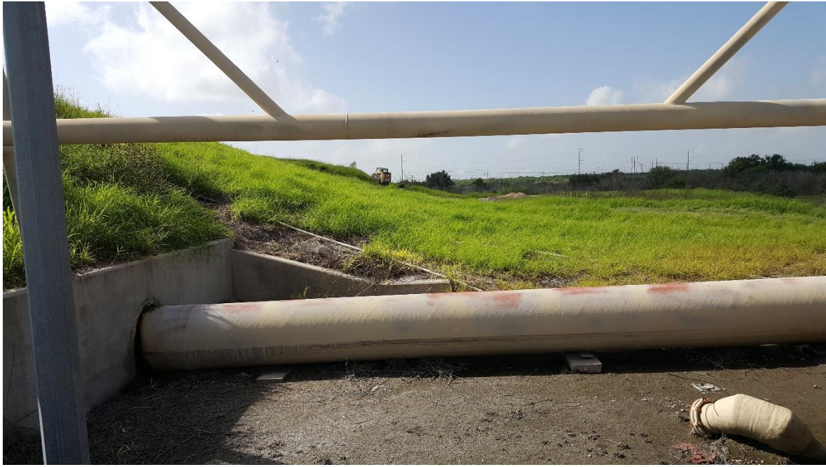
Photo 5 – View looking south at excess fill on west downstream slope by bulldozer.
