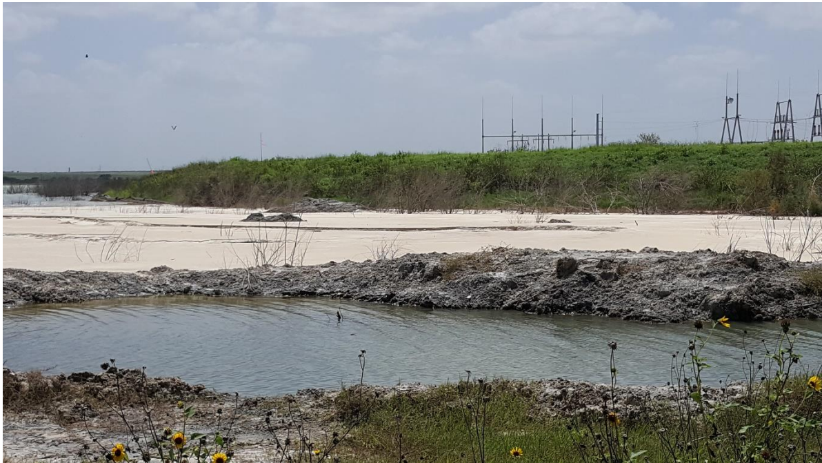
Photo 15 – View looking south from northeast corner of pond at bushes in pond and on upstream west slope.
