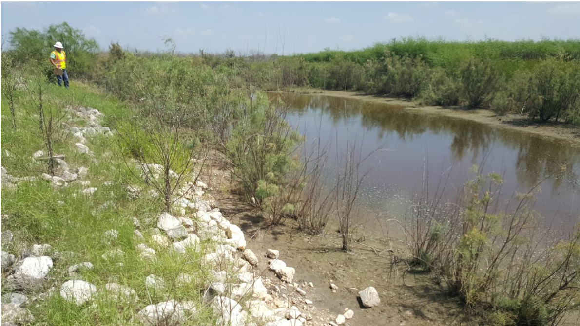
Photo 21 – View looking east at stone riprap and bushes on toe portion of south downstream slope and ponded water beyond slope toe.
