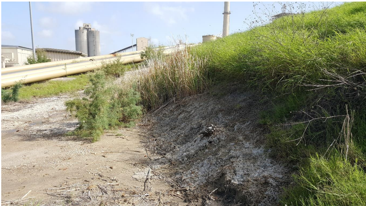
Photo 4 – Close up view of Photo 2 of cattails, stump in ground and steepened bottom part of slope.
