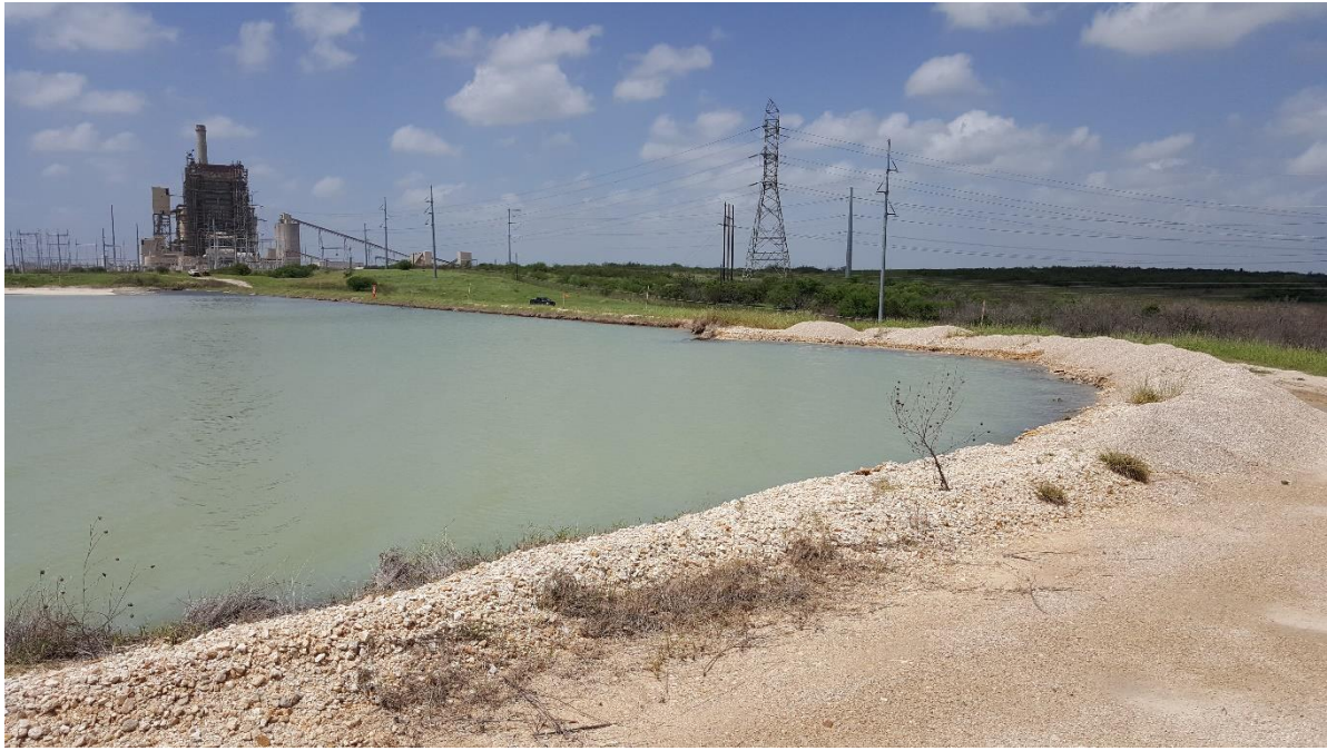
Photo 18 – View looking northeast at temporary dike along upstream crest in northeast corner of pond.
