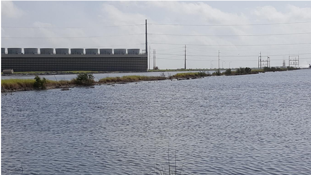
Photo 6 – View looking northeast at splitter dike with excessive bushes and grass.
