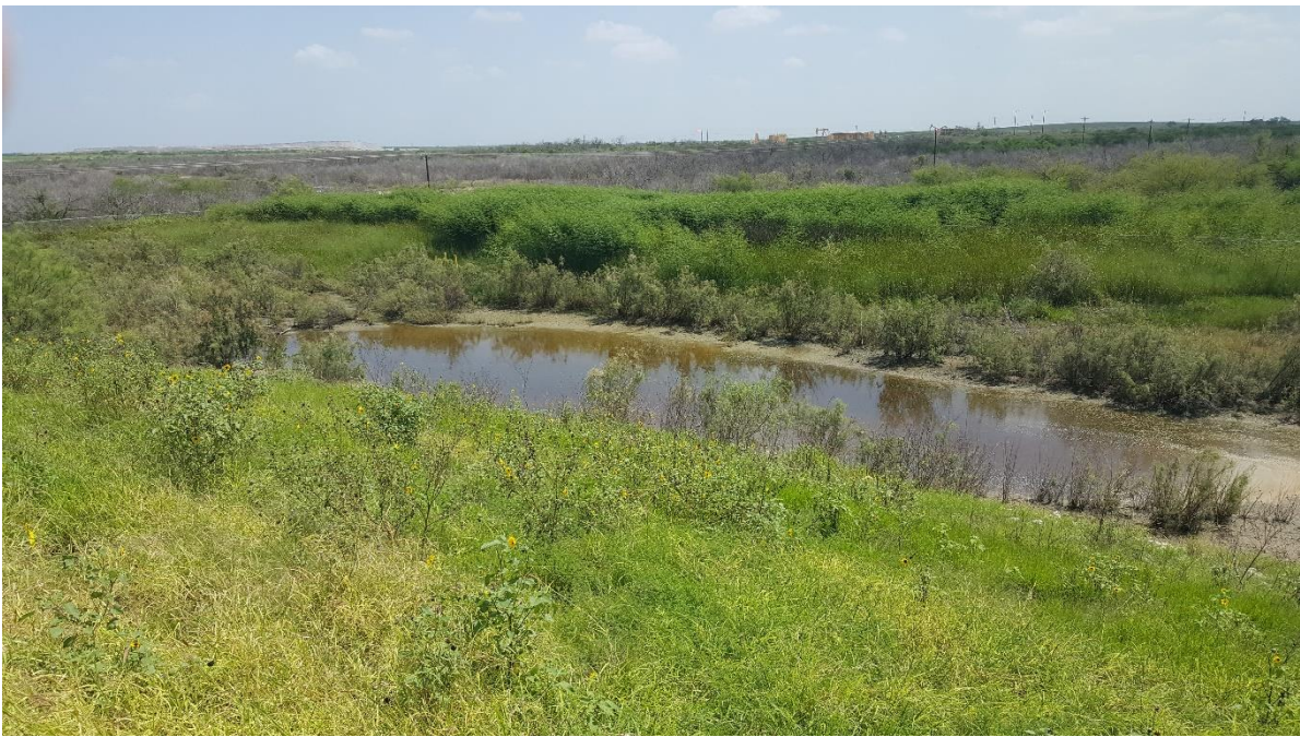
Photo 20 – View looking southeast from crest of south embankment at ponded water and bushes on downstream slope.
