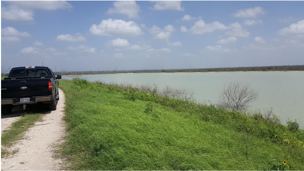
Photo 14 – View looking northeast at Equalization Pond from west side in central portion of bushes in upstream slope within pond.
