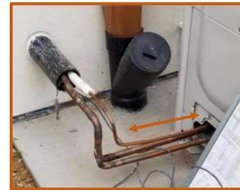
Main piping vertical elevation change
