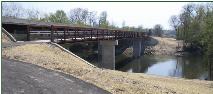
Bike trail bridge at Newtown Road
