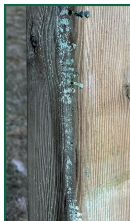
EFFLORESCENCES
