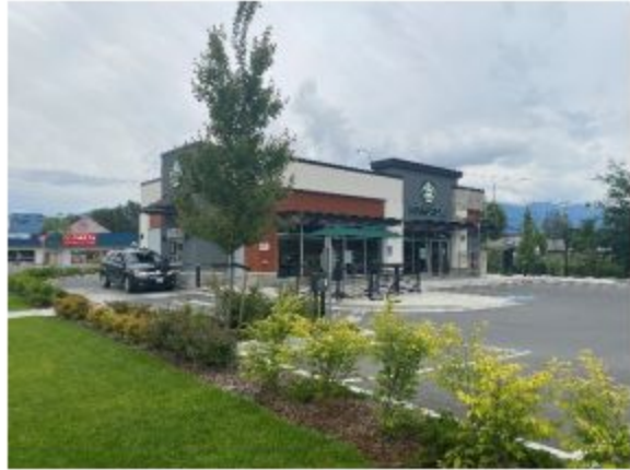
Subject Exterior Looking Southeast
