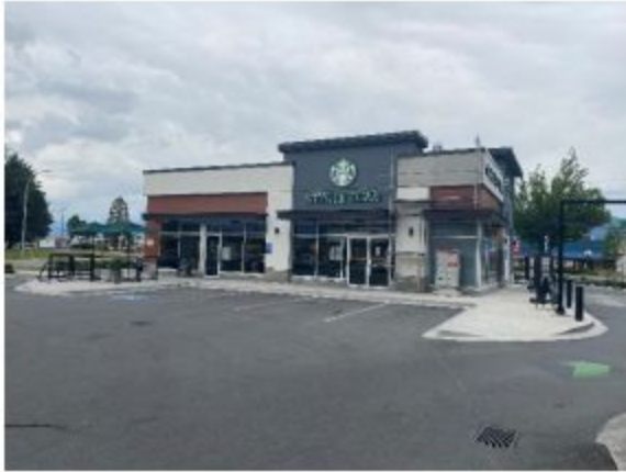
Subject Exterior Looking East
