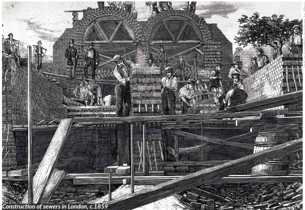
Construction of sewers in London, c.1859
