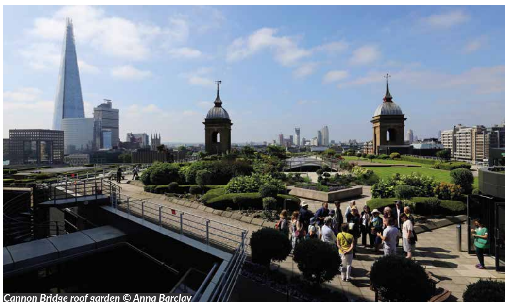
Cannon Bridge roof garden © Anna Barclay
