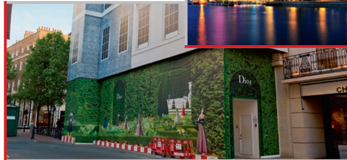
In a significant refurbishment and below ground expansion of Christian Dior's flagship store on New Bond Street, Newton products achieving both Type A and Type C waterproofing protection were integrated into the design at an early stage.
