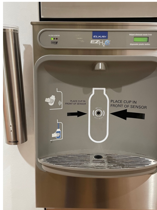
A stainless-steel water bottle refilling machine with a stainless-steel cup dispenser to its right, mounted on a white wall
