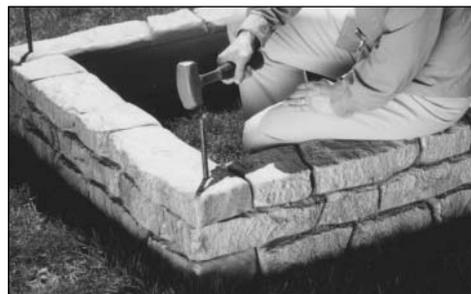
6. When you are finished, make sure the structure is where you want it to be, then hammer the steel spikes into the ground.
