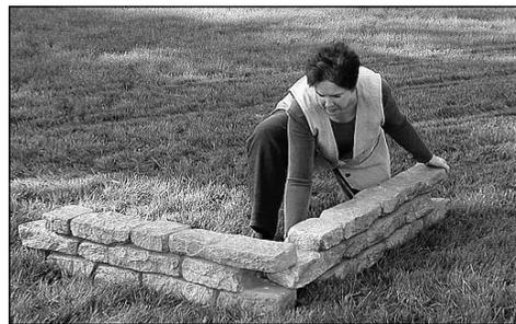
3. Interlock 2 sections together: WallRocks can be joined at either a 90-degree angle or as a straight line.
