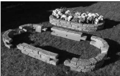
1. Select a layout configuration; some suggested layouts are on the previous page, or design your own. Lay the RockLock Wall System modules down in the rough locations.
