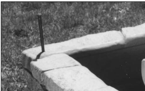
4. Insert a spike to secure the 2 sections together, but do not hammer into the ground until you are finished with the complete layout.
