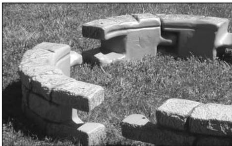
2. Make sure the rock-textured surfaces of the modules face the outside of the structure, with the rock-textured top surfaces facing up.
