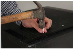
4. Insert the 4 plastic anchors into the 4 holes you drilled. You may need a hammer to secure the anchors.
