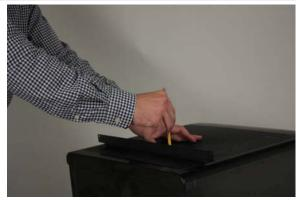
2. Remove the microwave and use the mounting bracket as a template to mark the 4 holes that will be drilled on top of the refrigerator.
