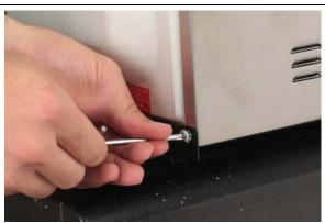
6. Use the Torx wrench to remove the two lower screws from the back of the microwave. Then, place the microwave against the bracket and secure the two screws with the Torx wrench.
