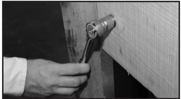
Removing skid from bottom of cabinet.
