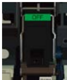
Class II panel with circuit breaker having a class II front face
