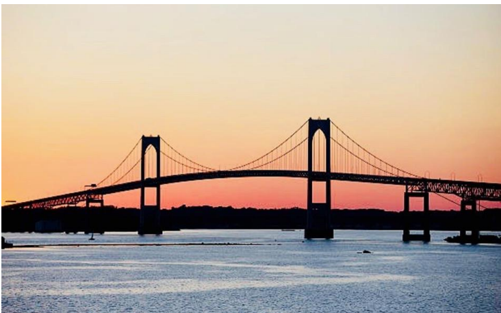
The Claiborne Pell Bridge, Newport, RI CORBIS VIA GETTY IMAGES
