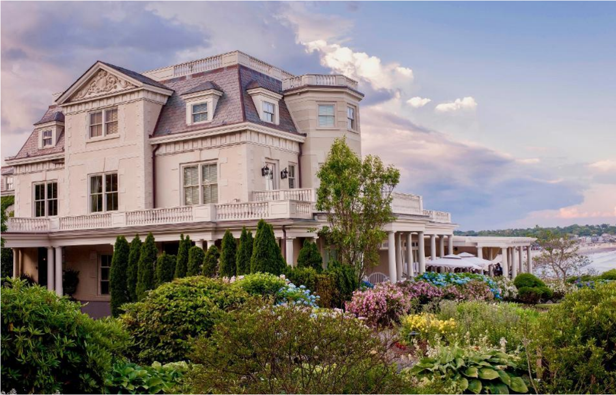
The exterior of the Chanler
