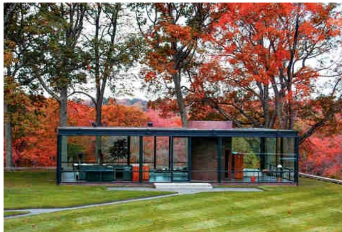
The Philip Johnson Glass House
