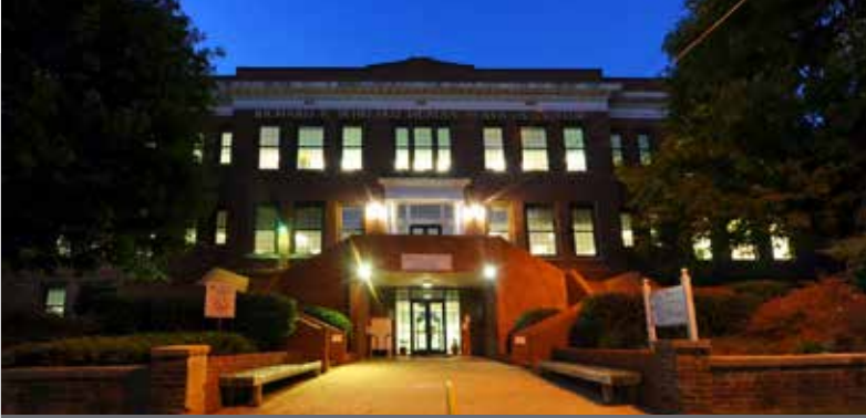
ORANGE COUNTY GOVERNMENT BUILDING: RICHARD E WHITTED HUMAN SERVICES CENTER
