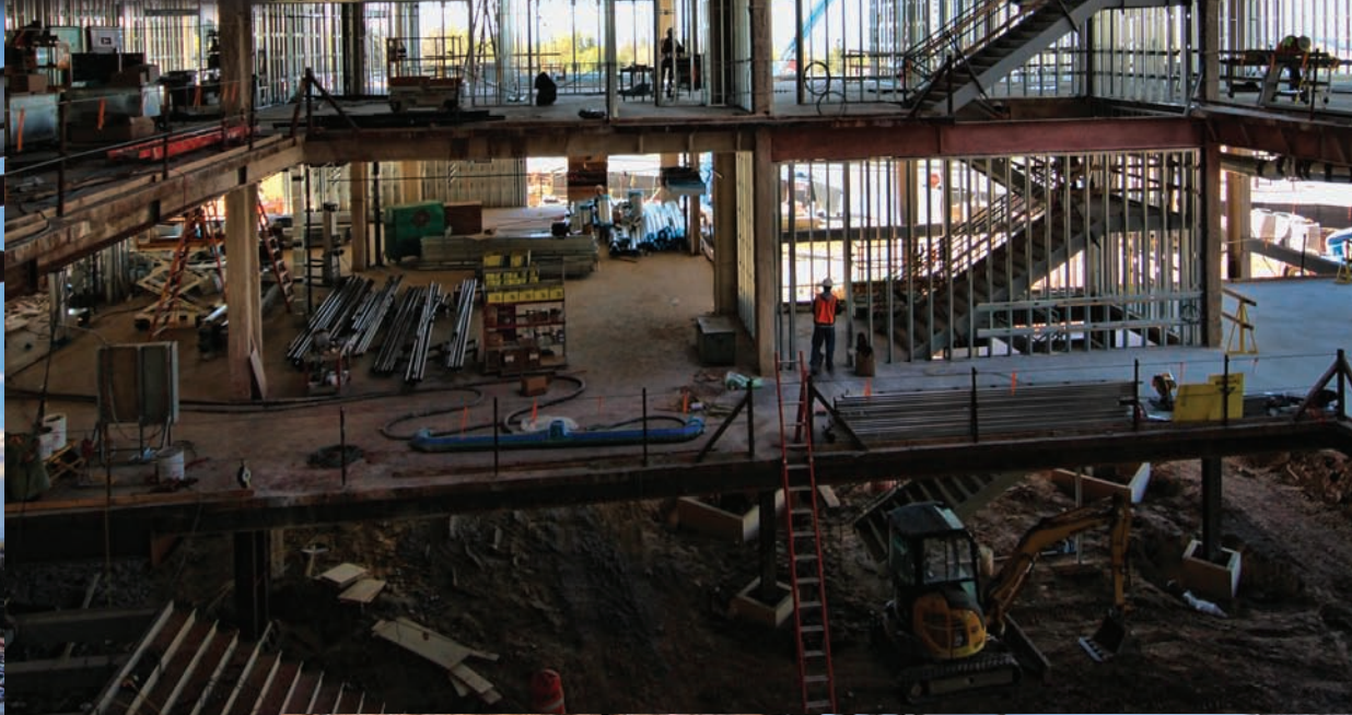
Construction of a gray water capture tank under the first floor. Water from the lavatories and showers sinks will be captured, treated and used to flush low-flow toilets in the building. Photo taken April, 2014
