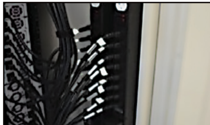
Side-by-side PDU mounting using 7" wide PDU mounting panel (Part No. XVMP024501)
