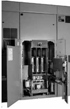
50L7 Vacuum Retrofit
