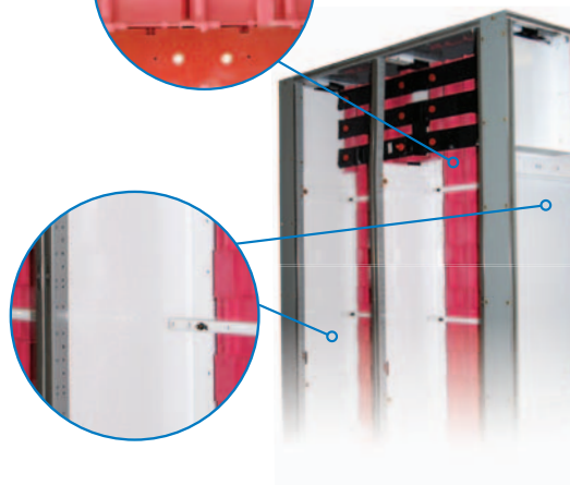
Rear View of Structure with Back and Side Sheets Removed
