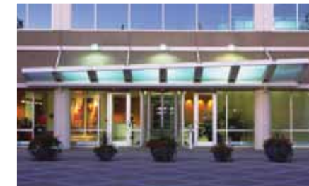
outdoor facility lighting
