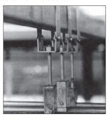
H-193 Hanger Rod supports conduit from G-962-D hanger. ASTM Class 2.
