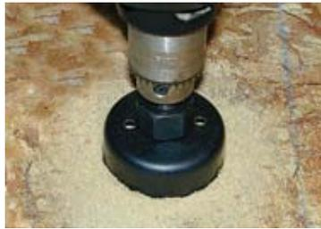
2. Drill hole in floor using hole saw.
