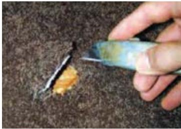
1. Cut a 2-3/8 in. hole through carpeting before using hole saw.
