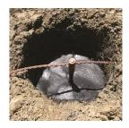
The nVent ERICO Hammerlock irreversible mechanical connection connects the grounding conductor to the ground rod. Machined from highly conductive copper, the state-of-the-art Hammerlock provides a low resistance connection designed to withstand ground fault currents and lightning transients. The connector's mechanically rugged design will help ensure that the highest level of performance is maintained for many years after the connection has been buried in the harsh underground environment.
