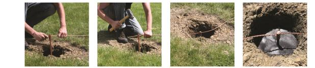
The nVent ERICO Hammerlock irreversible mechanical connection connects the grounding conductor to the ground rod. Machined from highly conductive copper, the state-of-the-art Hammerlock provides a low resistance connection designed to withstand ground fault currents and lightning transients. The connector's mechanically rugged design will help ensure that the highest level of performance is maintained for many years after the connection has been buried in the harsh underground environment.
